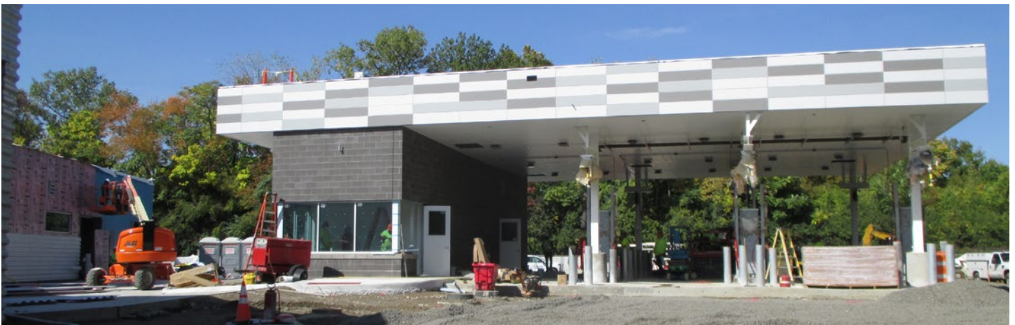
COTA FIELDS AVE UNDER CONSTRUCTION
