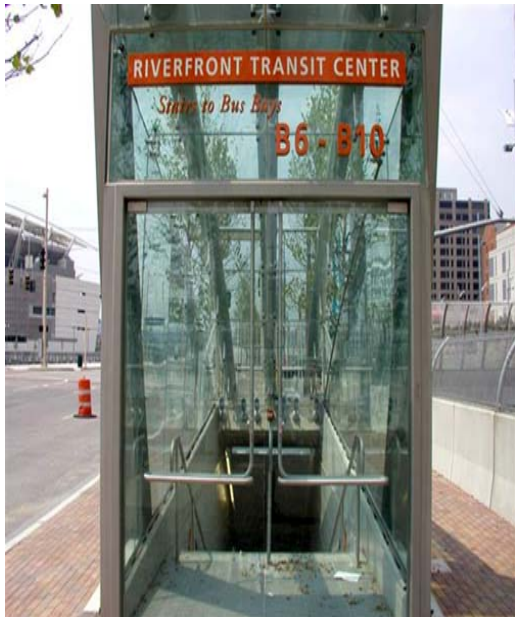
Transit Center Sidewalk Entrance
