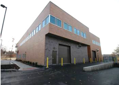
View of Cincinnati Public Works Rear Entrance
