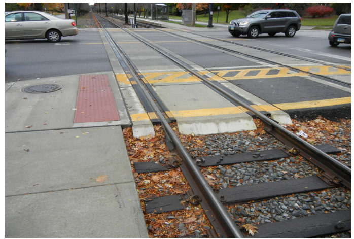
GCRTA ADA Track Crossing
