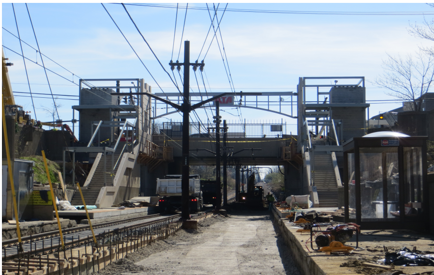
HWH Observing Construction of Lee Van Aken Station & Track Adjustment
