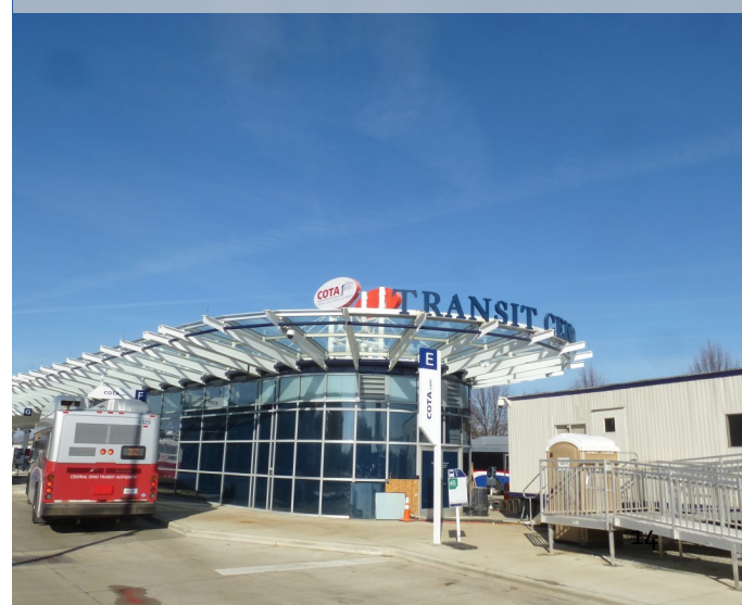
Easton Transit Center Renovation, COTA, Columbus, OH
