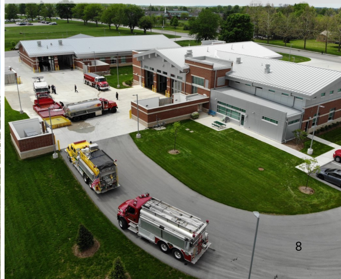
Plainfield Fire Station & Headquarters Campus
