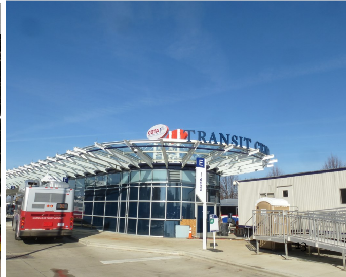
Easton Transit Center Renovation, COTA, Columbus, OH
