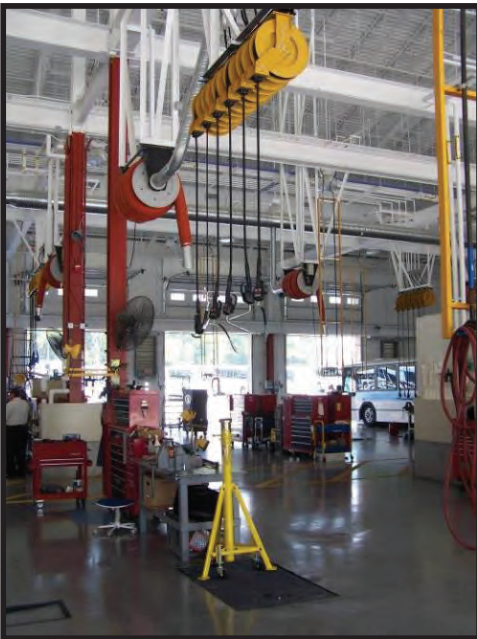
WSP specializes in developing functional and efficient spaces such as this repair bay in the Chapel Hill Town Services Center.
