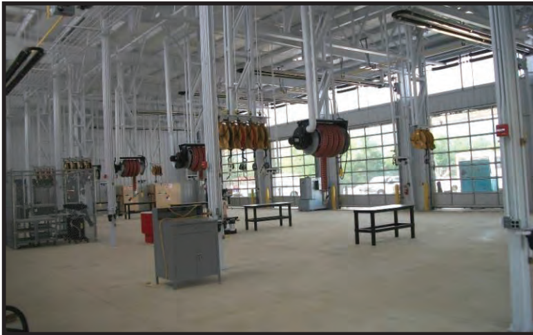
WSP provided services for this maintenance facility, allowing greater access to transit vehicles being serviced.
