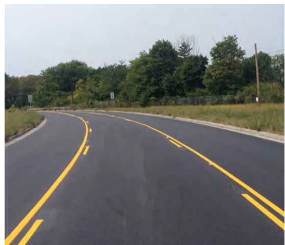
Oxford State Road Reconstruction Project
