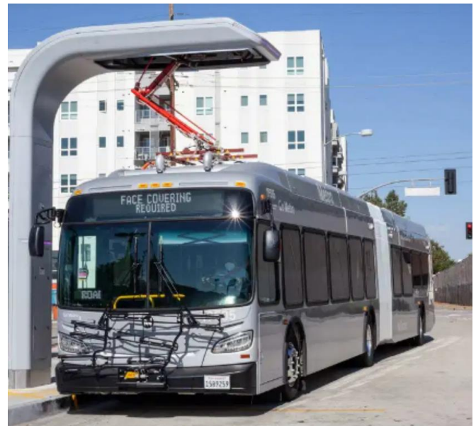
Figure 2-3. On-Route Overhead Charging, Los Angeles Metro
