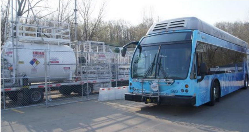
Figure 2-12. Mobile Hydrogen Fueling Station, Canton, Ohio
