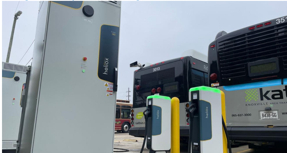
Figure 2-2. Dispenser and Charger Cabinets, Knoxville Area Transit
