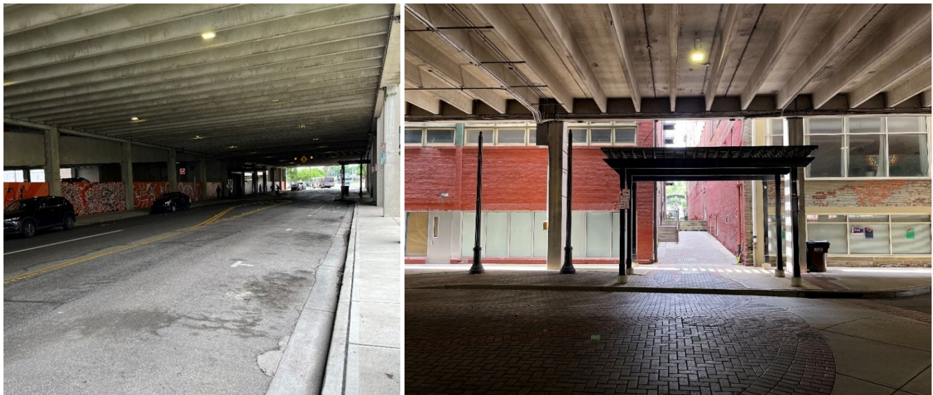
Figure 4: Existing Conditions at Market Street Station
